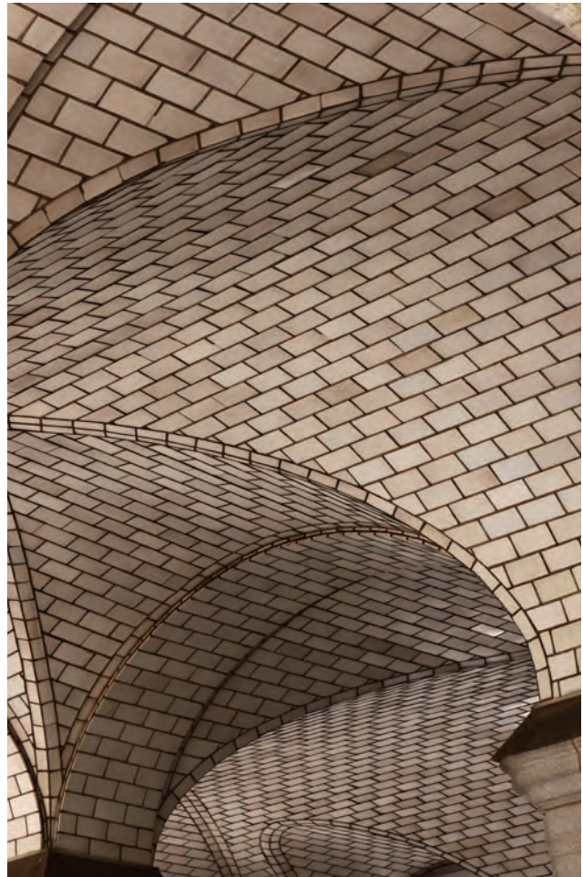
Vaulted ceiling with Guastavino tiles, Manhattan Municipal Building, New York City, completed in 1914.
