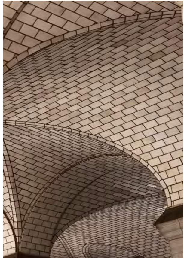
Vaulted ceiling with Guastavino tiles, Manhattan Municipal Building, New York City, completed in 1914.
