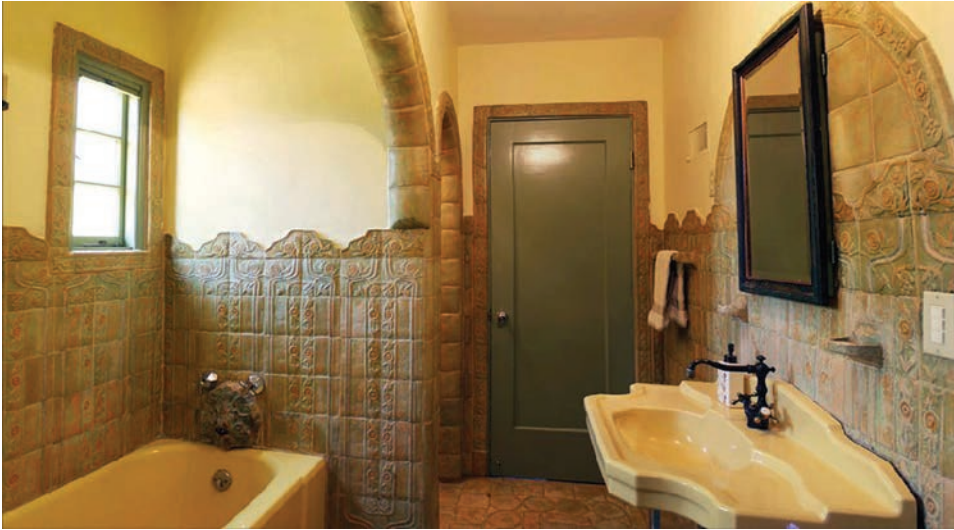
Tiles by Handcraft Tile Co. of Milpitas, California adorn this 1937 Spanish Colonial residence in San Jose.
