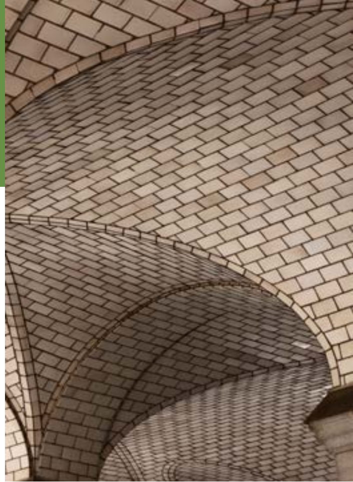
Vaulted ceiling with Guastavino tiles, Manhattan Municipal Building, New York City, completed in 1914
